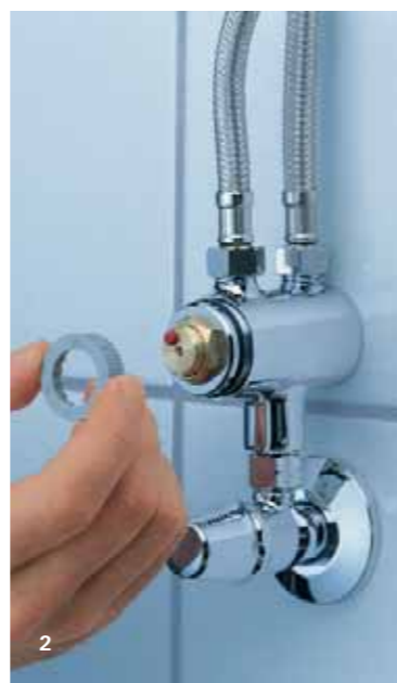
1 Temperature adjustment using Allen key 2 Re-attach scale ring
