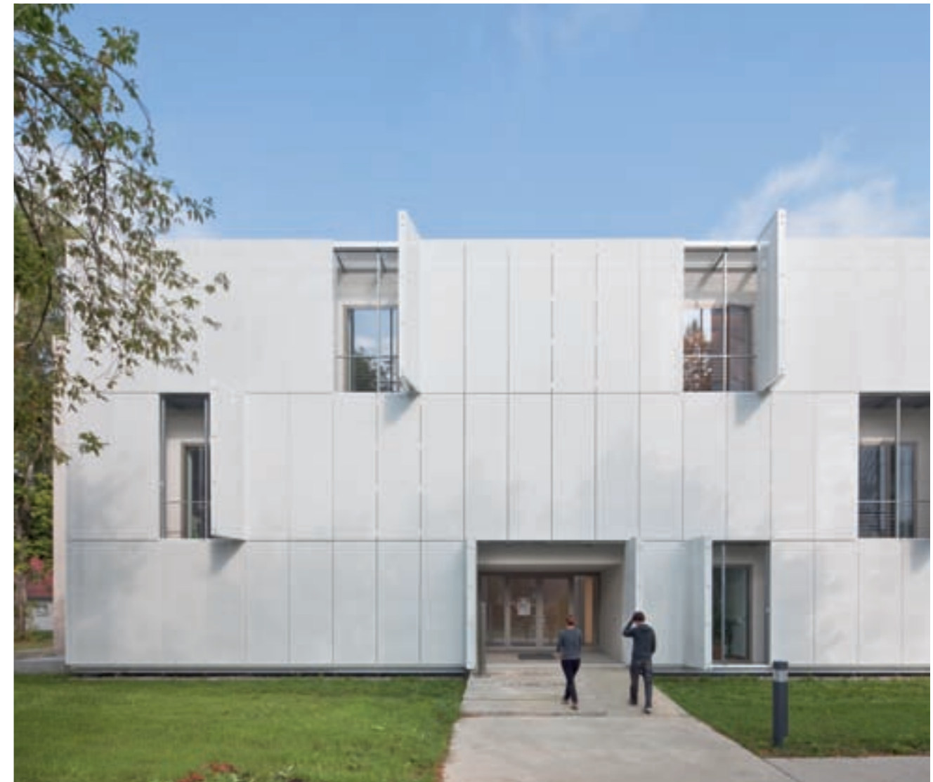
The front consists of white coated expanded metal which serves as a sunscreen and lets evenly filtered light stream through its fine pores into the workspaces.
